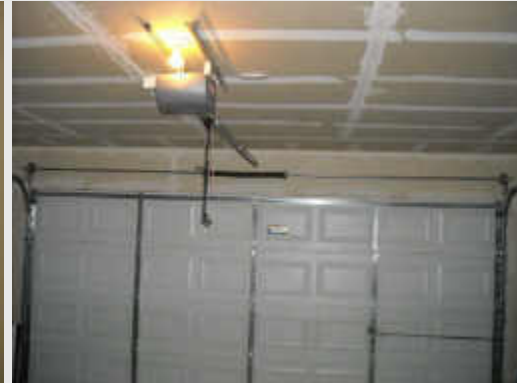
New Garage Door opener for this double garage
