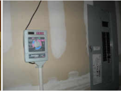
Automatic Lawn Sprinkler System to help with the worry free yard
